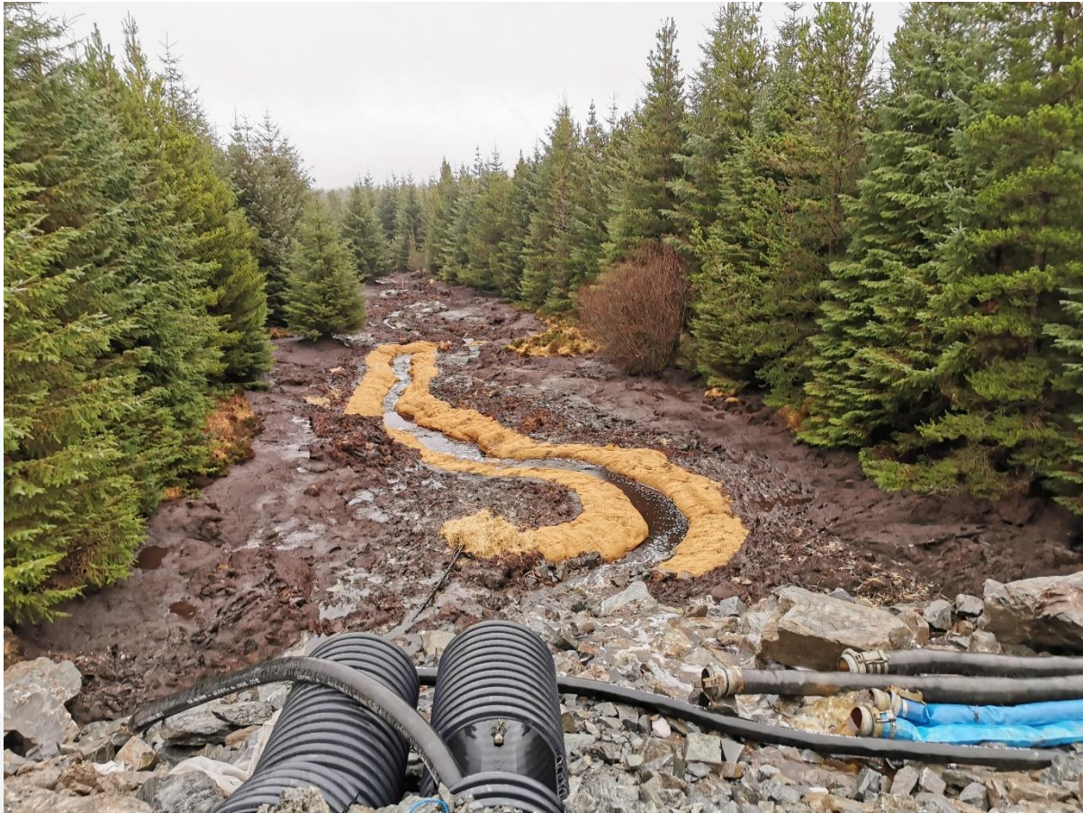
Plate 3 Coir matting installed on the Shruhanganrve downstream of Wall 1.
