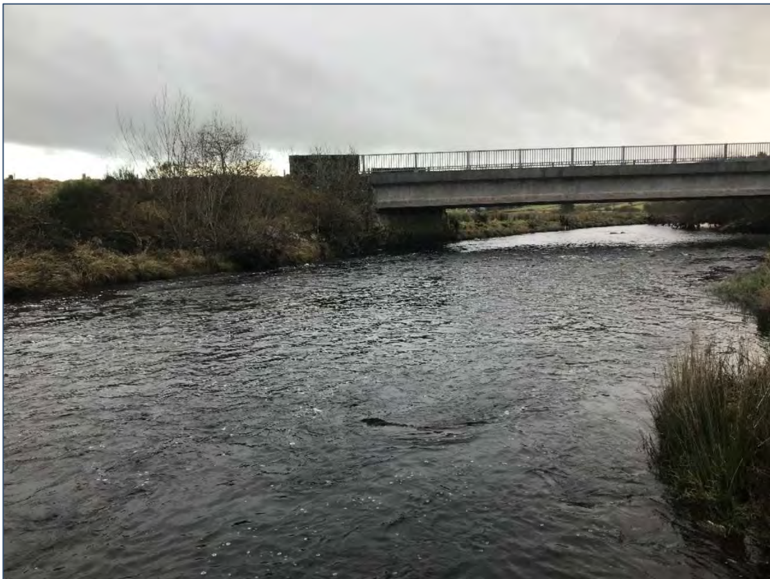
Plate 3-7. Mourne Beg River at Survey Section Three
