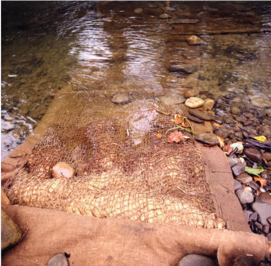
Plate 4 Sedimat installed on stream bed to trap suspended sediment through upper layer of jute mesh and lower layers of wood wool.
